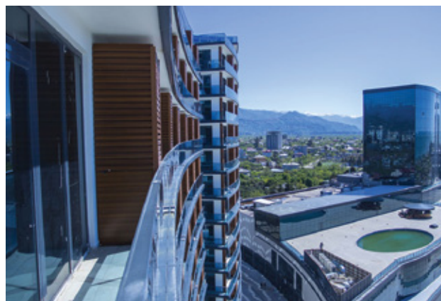
METRO CITY APARTMENTS
